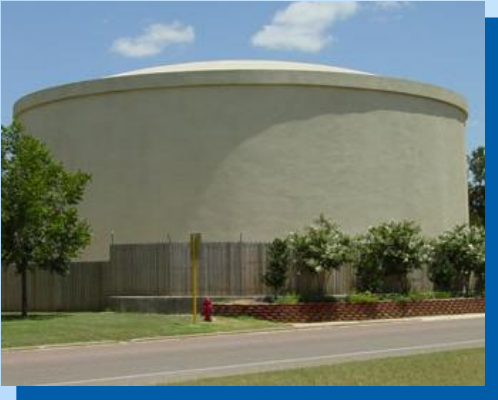
Ground Storage Tanks
