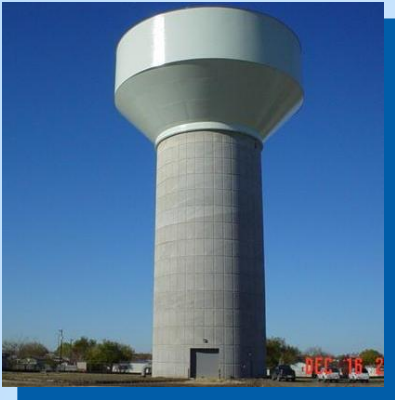
Elevated Storage Tanks
