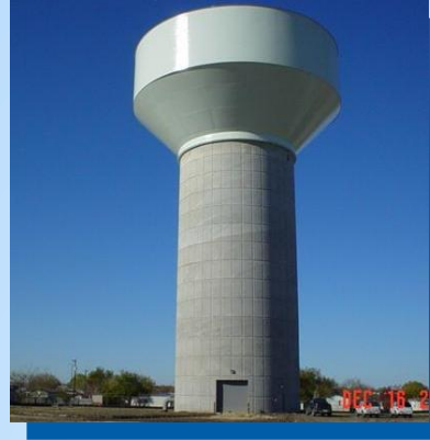
Elevated Storage Tanks
