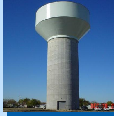
Elevated Storage Tanks
