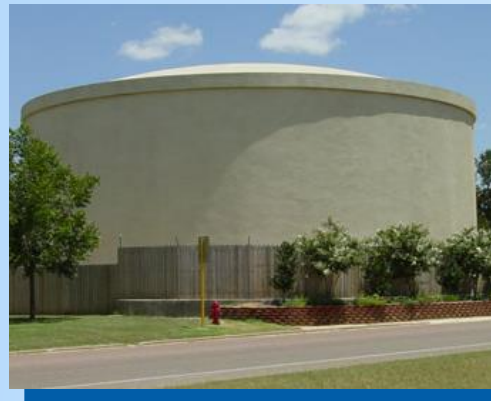
Ground Storage Tanks
