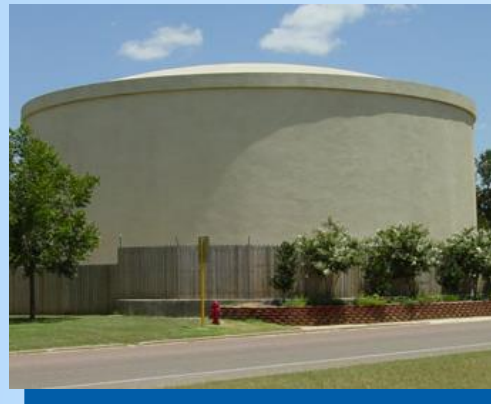
Ground Storage Tanks
