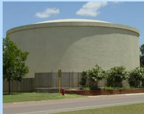
Ground Storage Tanks
