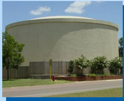
Ground Storage Tanks
